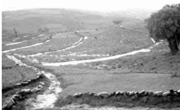
Graded bund and ditch below with drainage channels. Excess water needs to be drained and channelled without causing damage. Anjeni, Ethiopia. (Photo: Hans Hurni)
