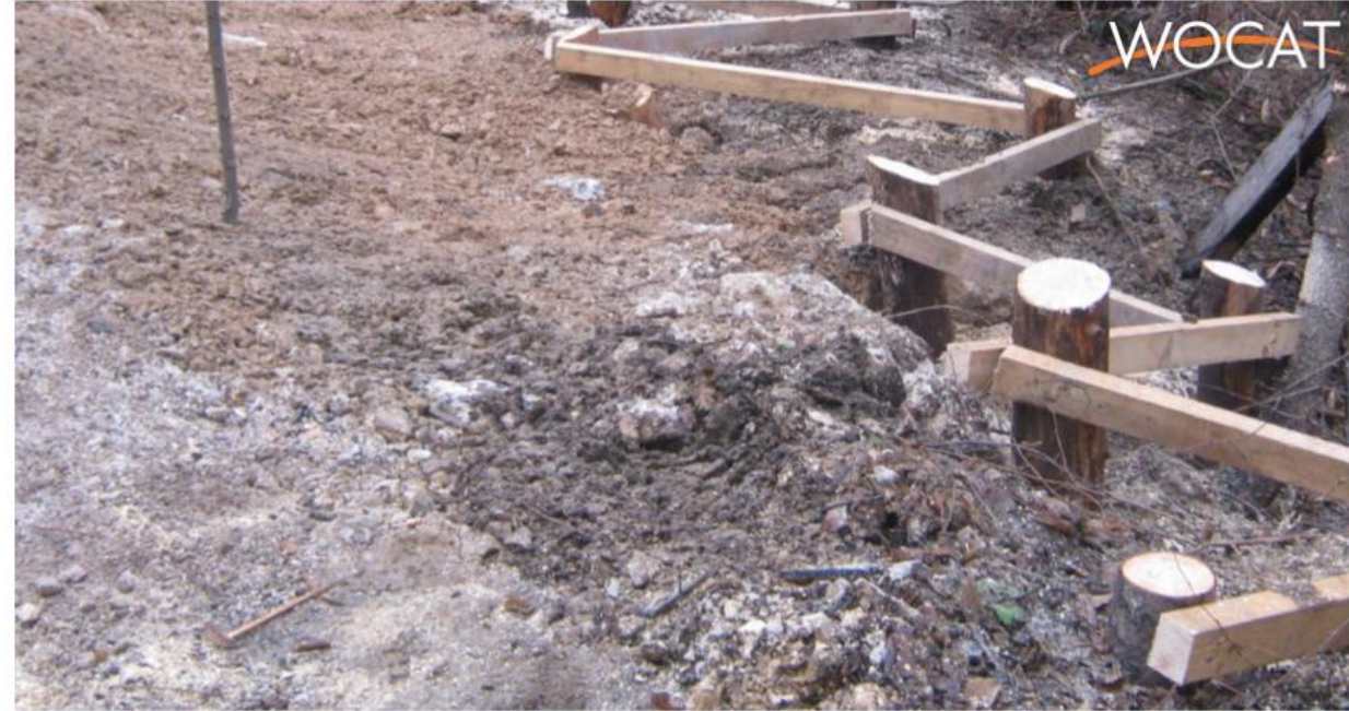
Wooden poles used to stop movement of landslide (Photo archive of the Kladanj municipality)
