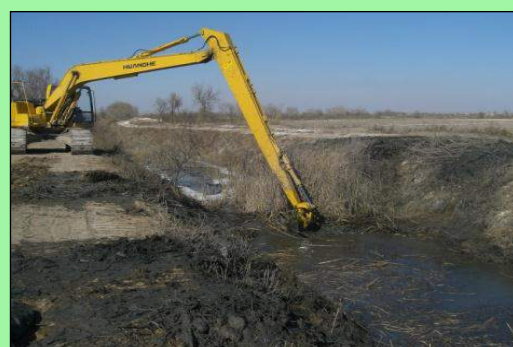
Figure 2. Cleaning a collector.
