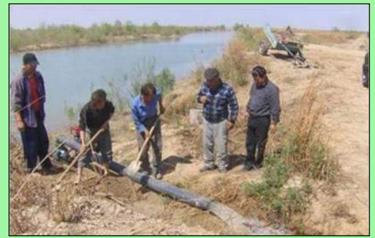
Figure 1. Tenants of communal forestry, inhabitants from near-tugai auls (villages), install pump for organization of irrigation of saplings (photo by: Aybergenov B.)
