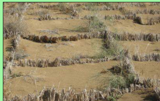
Figure 1. The established cellular mechanical protection with the planted seedlings of Haloxylon persicum (photo by Nikolay Zverev)
