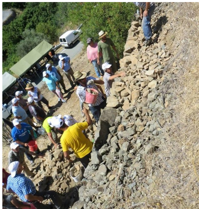
Participatory rehabilitation of dry-stone terraces (Christos Zoumidis)
