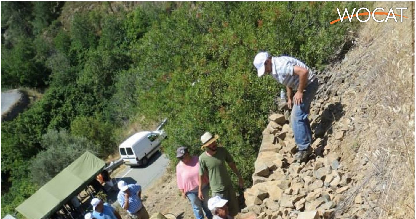
Participatory rehabilitation of dry-stone terraces (Christos Zoumidis)
