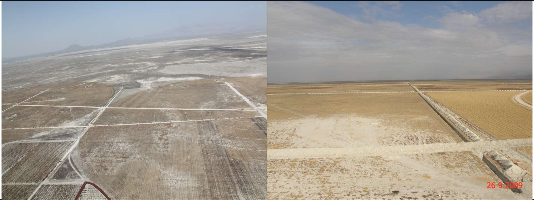
Photo 23. An effective drainage system is very important in the UNSPED farm because soils are saline and have a very low permeability. In the irrigated agriculture, without excess water drainage salinity becomes a big problem. The image on the left shows the pattern of built drainage lines with white colors where salts concentrate. Excess waters are being drained to the Akgöl depression, where is the lowest elevation in the subbasin, which can be traced up with photo above left..
