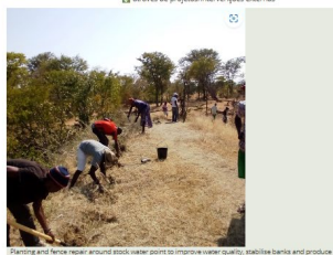
Planting and fence near around Biebe water point to improve water quality, stabilize banks and protect water. (Project RETSA)
