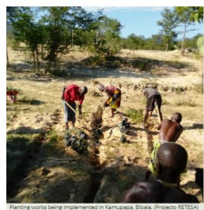
Planting work being implemented in Kamupula, Biebe. (Project RETSA)
