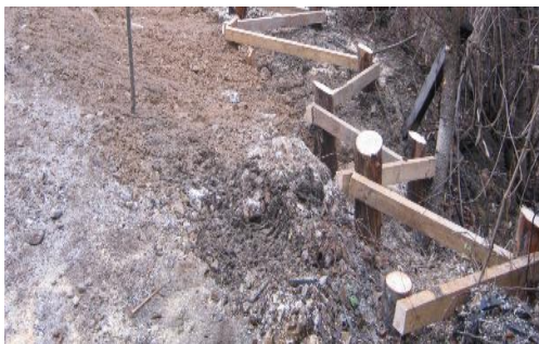
FIGURE 44. Connecting adjacent piles with wooden laths (Photo: Archives of the Municipality of Kladanj)
