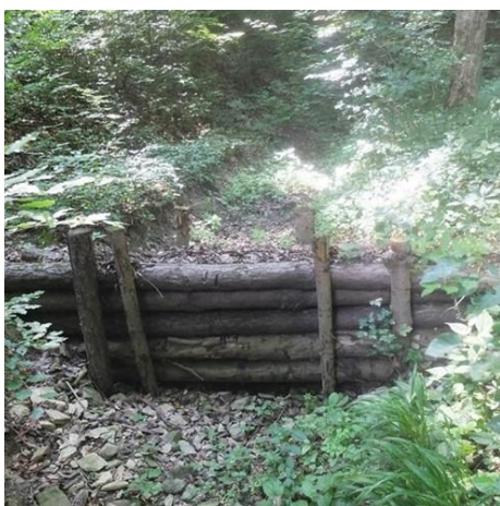
FIGURE 56. Wooden dam during the dry summer period
