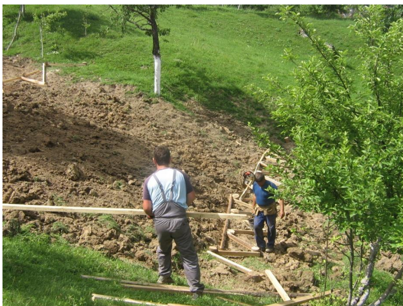
FIGURE 43. Installation of timber pile formation (Photo: Archives of the Municipality of Kladanj)
