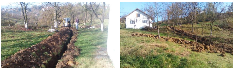
FIGURE 52. Installation of the „herringbone“ drainage system in the area of Omazići - Husanovići (Photo: S. Husanović, 2019)
